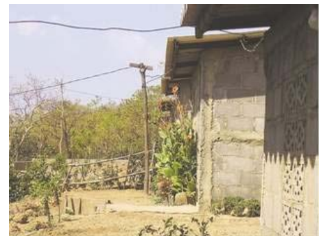
These homes in the Tuma community in rural Nicaragua are part of Rainbow Network's housing program. The homes cost about $2,500 to build, and homeowners pay as little as $6 per month on an interest-free loan. (Rainbow Network)
